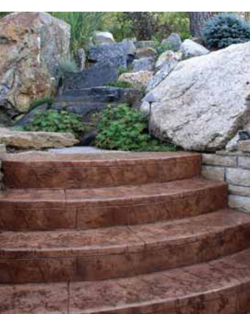
Stamped concrete steps lead to a patio made of the same material, which features the fireplace and kitchen.
