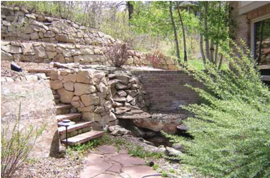
Part of the backyard renovation project was to remove the crumbling rhyolite walls and stagnant water feature behind the home.
